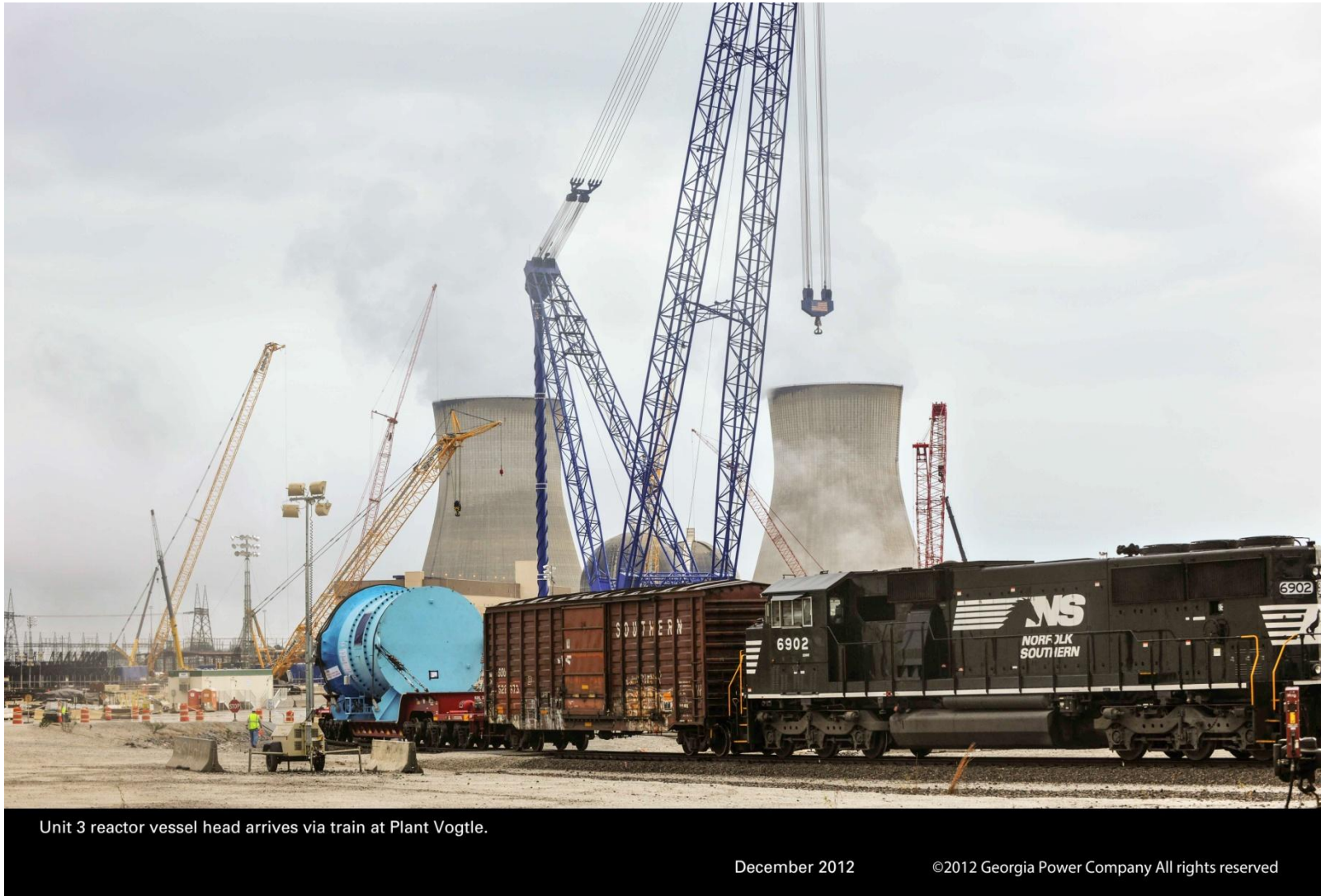
Photo 10 – Unit 3 Reactor Vessel Head Delivery
